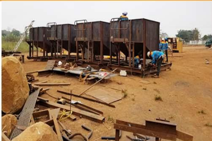
FABRICATION AND INSTALLATION OF STALKER TANKS
