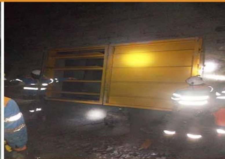
FABRICATION AND INSTALLATION OF LOUVER DAMPERS
